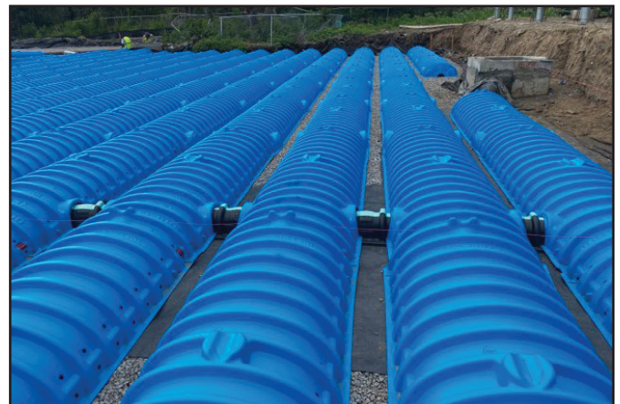
Shown: CULTEC HVLV SFCx2 Feed Connector inserted into side portals of CULTEC chamber.
