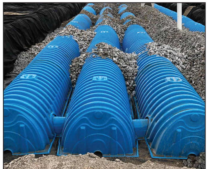
Shown: CULTEC HVLV FC-24 Feed Connector inserted into side portals of CULTEC chamber.
